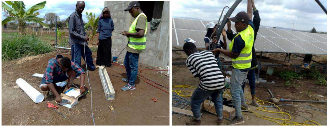
Figure 14: Shows ToTs participating in pump installation during ToTs technician training.
