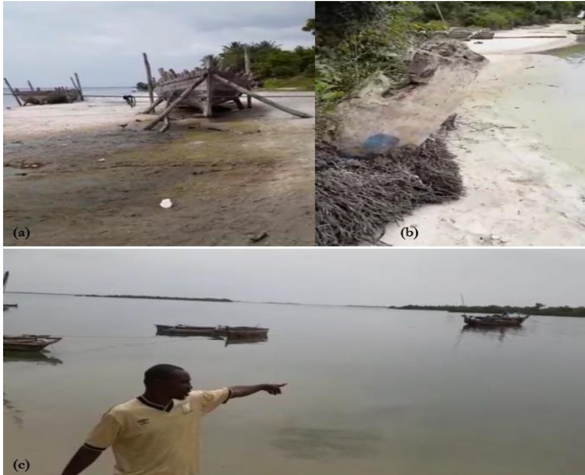
Figure 20: Massive land loss and damages at Mlingotini village in Bagamoyo District
