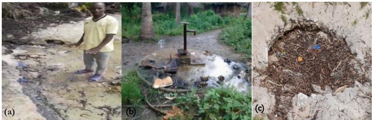
Figure 22: Loss and damage evidences experienced in the study area
